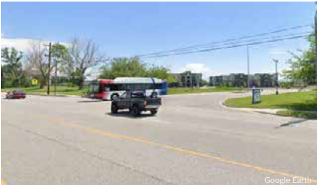
Existing Conditions - Clearfield Station Entrance
